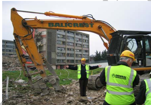
Former estate on Tanner Street undergoing demolition
